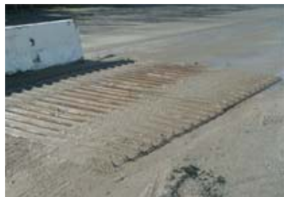
Rumble grates help dislodge stones from tire treads but require frequent cleaning
